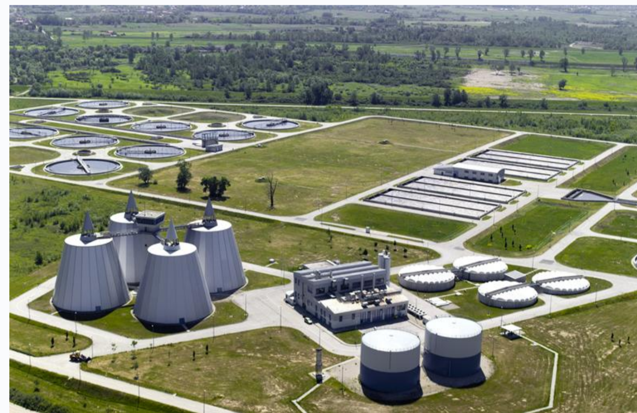
Figure 1: Municipal wastewater treatment plant of the City of Zagreb.
